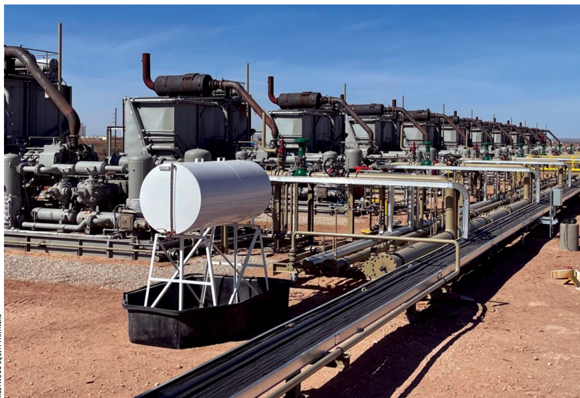
The Herradura compressor station is Crestwood's newest station, with capacity of more than 100 MMcf/d. It was commissioned in April.
