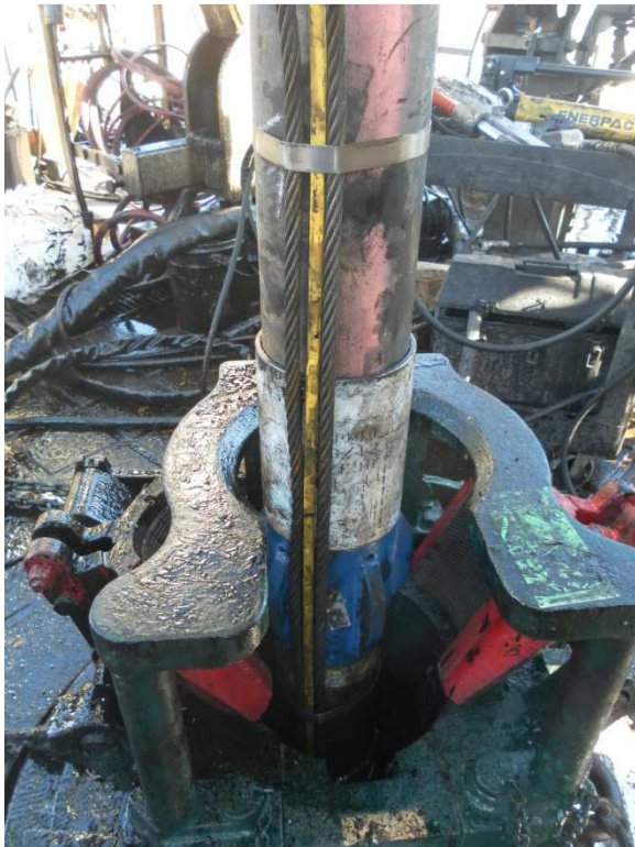
Fig. 11. The fiber line is banded to casing along with 1/2" inch braided steel cables paralleling on each side. The blue centralizer is locked in place beneath the casing coupling.
