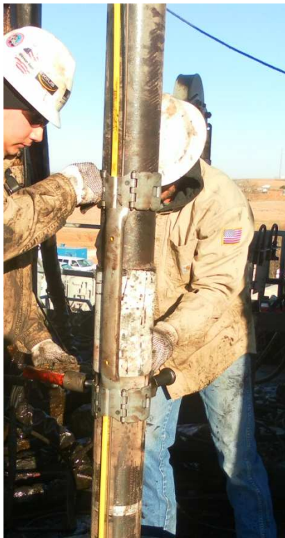
Fig. 11. Service company personnel install a cross coupling clamp.
