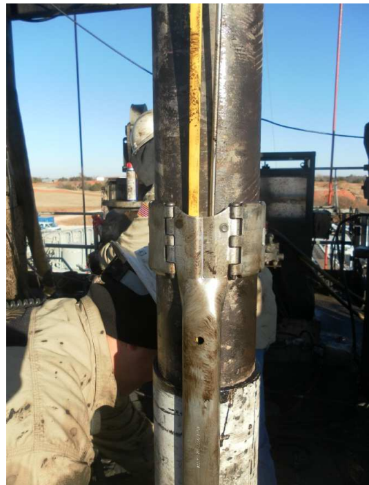
Fig. 12. A cross coupling clamp holds the yellow fiber optic line and the BHP gauge line to the 5-1/2" casing.
