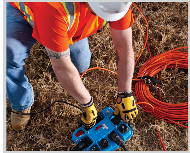
The temporary deployment of cables and sensors leaves minimal disturbance to property and the environment.
