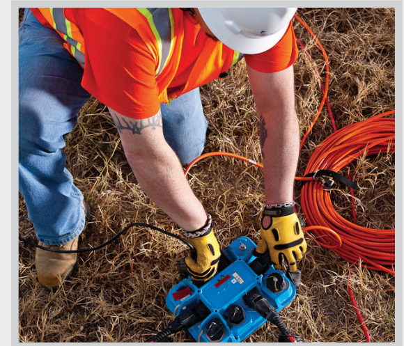
The temporary deployment of cables and sensors leaves minimal disturbance to property and the environment.
